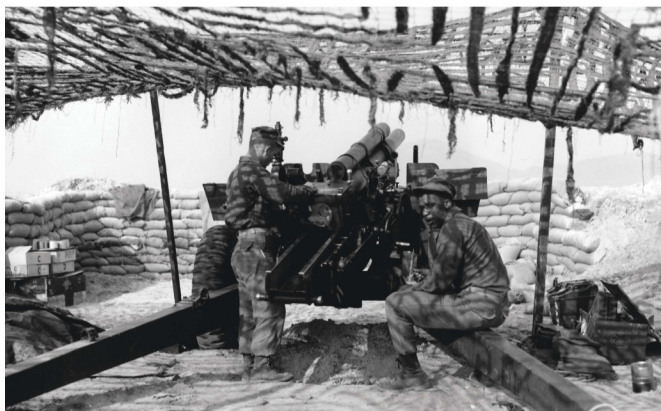
Above: Marine 105 mm howitzers provided an umbrella of steel around the perimeter of Da Nang Air Base. This firing position, similar to others, is protected by earthen works supported by sandbags and nets overhead for camouflage. (Photo by SSgt Batchelor, USMC)
