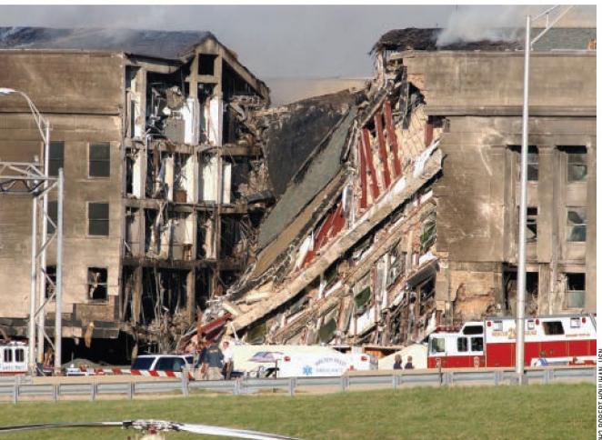
A portion of the Pentagon collapsed when the fire from the impact of American Airlines Flight 77 weakened parts of the western wall.
