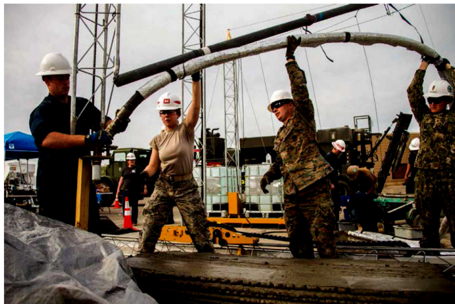
7th Engineer Support Battalion Marines and Naval Mobile Construction Battalion 5 used the automated construction of an expeditionary structure printer to conduct 3D printing. (Photo by LCpl Betzabeth Galvan.)
