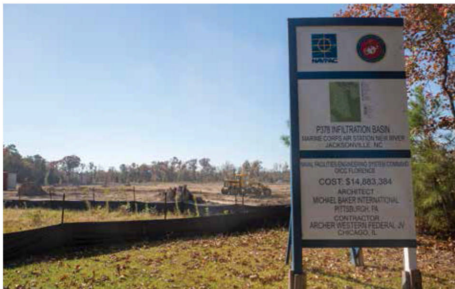
This water infiltration basin will provide MCAS New River with 190 acres of impervious area and will be able to handle the first two inches of storm water runoff. This decreases the need for stormwater ponds on the flightline, reducing Bird/Aircraft Strike Hazard (BASH) concerns by eliminating the bird habitat. (Photo by Cpl Christian Ayers.)
