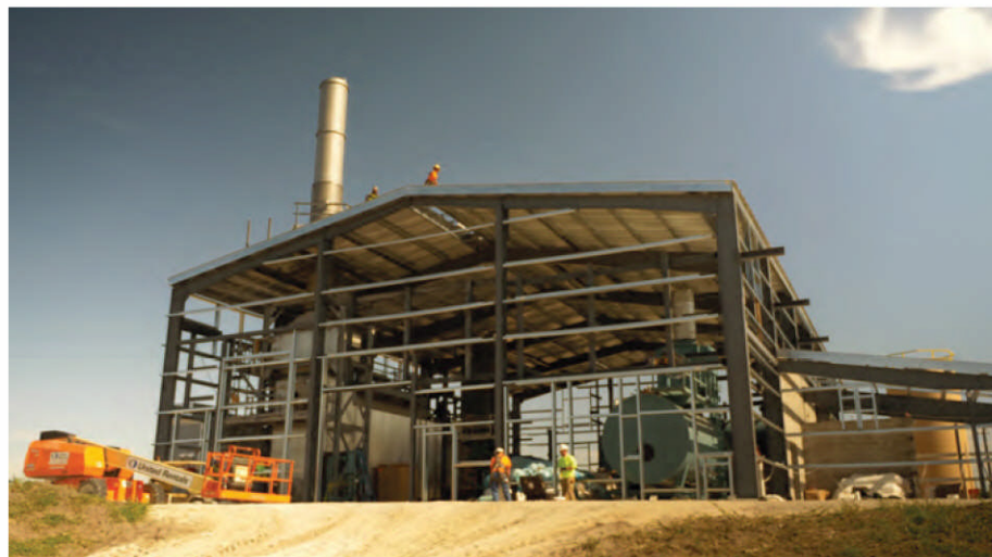
The new cogeneration (CHP) plant at MCRD Parris Island under construction in July 2018. (Photo by author.)
